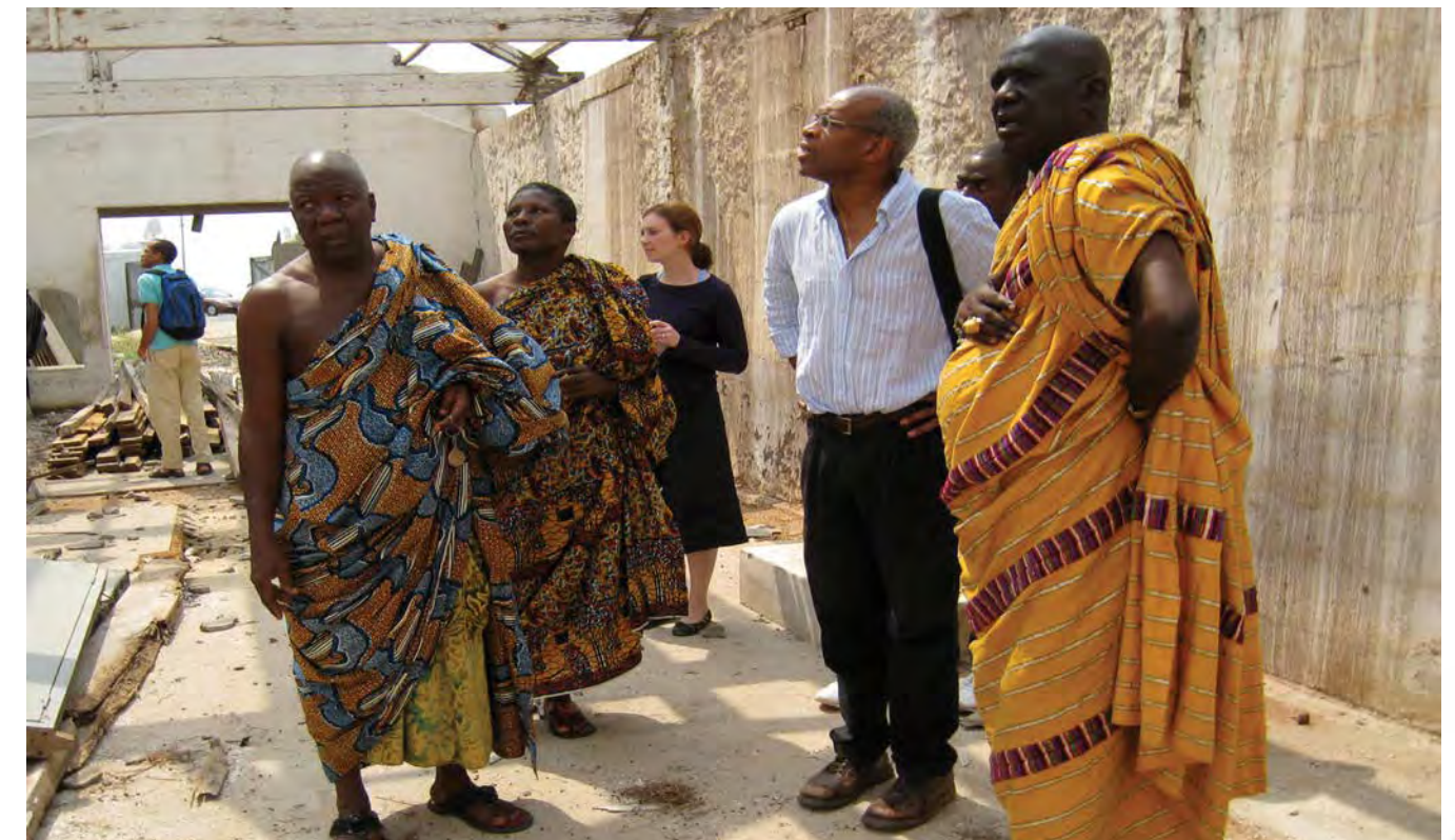
Surveying Gothic House with the Omanhene Chief of the Oguaa Traditional Council Left: A Sketch of the Proposed Renovations of Gothic House
