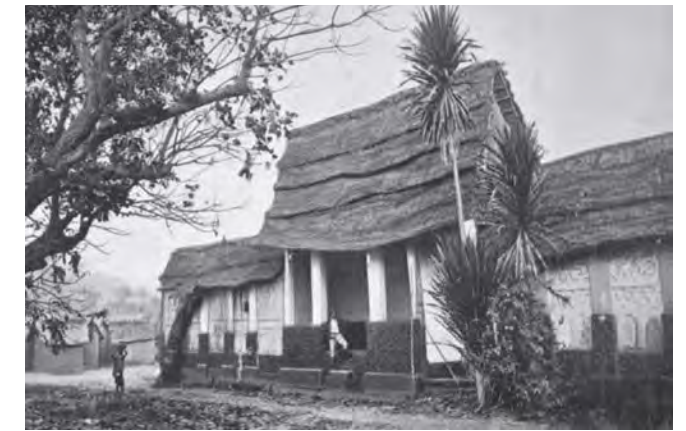
Original Pitched Roof, ~1888-1896
