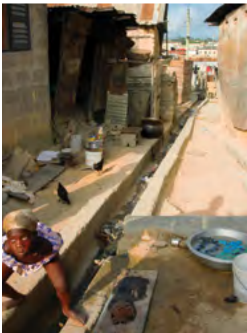
Fig. 18 Open sewage canal in the Zongo.
