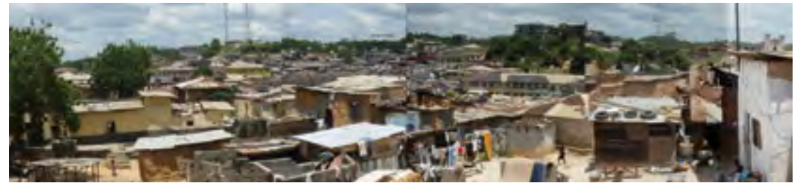
Fig. 9 Urban condition – Zongo.
