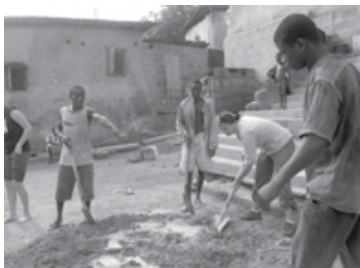
Fig. 33 Mixing of sandcrete.
