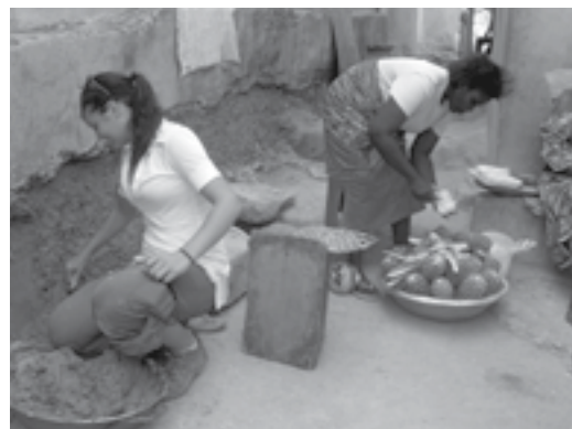
Fig. 34 Application of landcrete.
