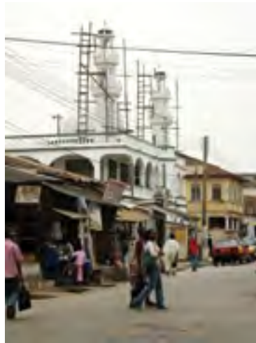
Fig. 5 Mosque under construction.
